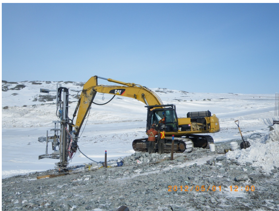
Photo 3: Inclinator installation at ND-IN-120-1 complete. Retrieval of outer steel casing lost in borehole ND-IN-120-3 in progress.
